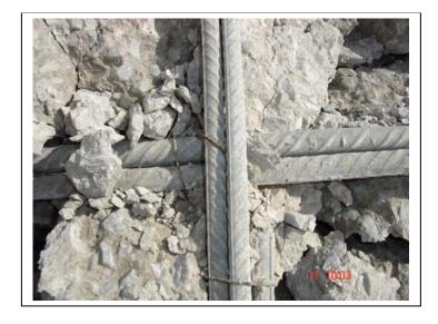
Condition of exposed hot dip galvanized reinforcement found during the demolition of the 20 year old approach stairway. With isolated exceptions, the hot dip galvanized reinforcing shown, in this photograph, is typical of 98% of that inspected.
