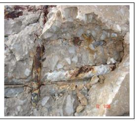
Isolated red rust was found, usually associated with minimum concrete cover and/or mechanical damage to the concrete cover.
