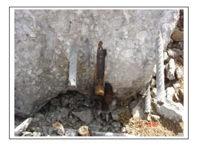
This photograph shows two uncoated reinforcing bars that were used in the stairway without being hot dip galvanizing. The corrosive attack is clearly evident, while the hot dip galvanized bars located alongside are performing with complete satisfaction.
