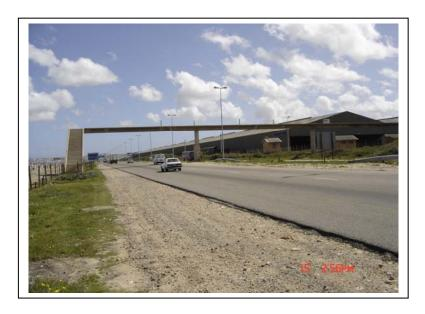
The site of the 40-year-old pedestrian bridge (No B776) that was demolished in April 2005. It was established that hot dip galvanized reinforcement was used in the approach stairway, which was on the sea facing side, indicated on the left of the photograph, with the sea some 50 meters further left. This stairway was part of a refurbishment of the seriously corroding structure in 1985.
