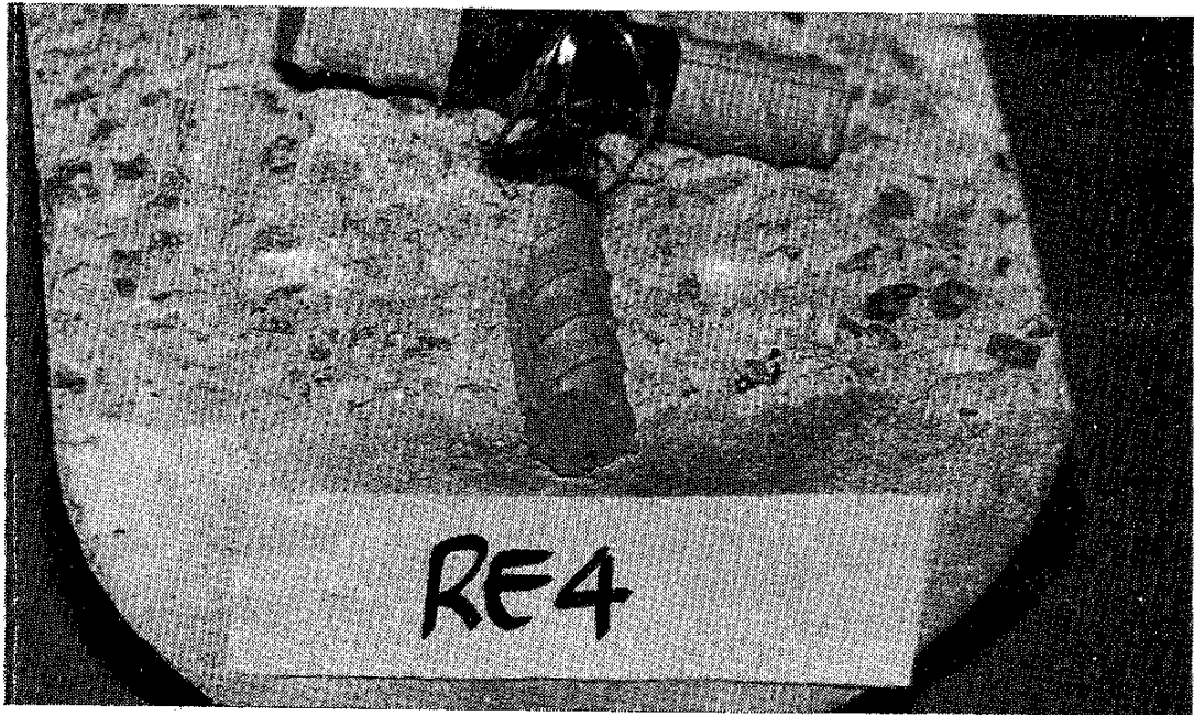
Plate 3: Sample RE4: Epoxy Coated Steel - Atmosphere - 41 Days. Localized corrosion at repaired exposed end of longitudinal bar.
