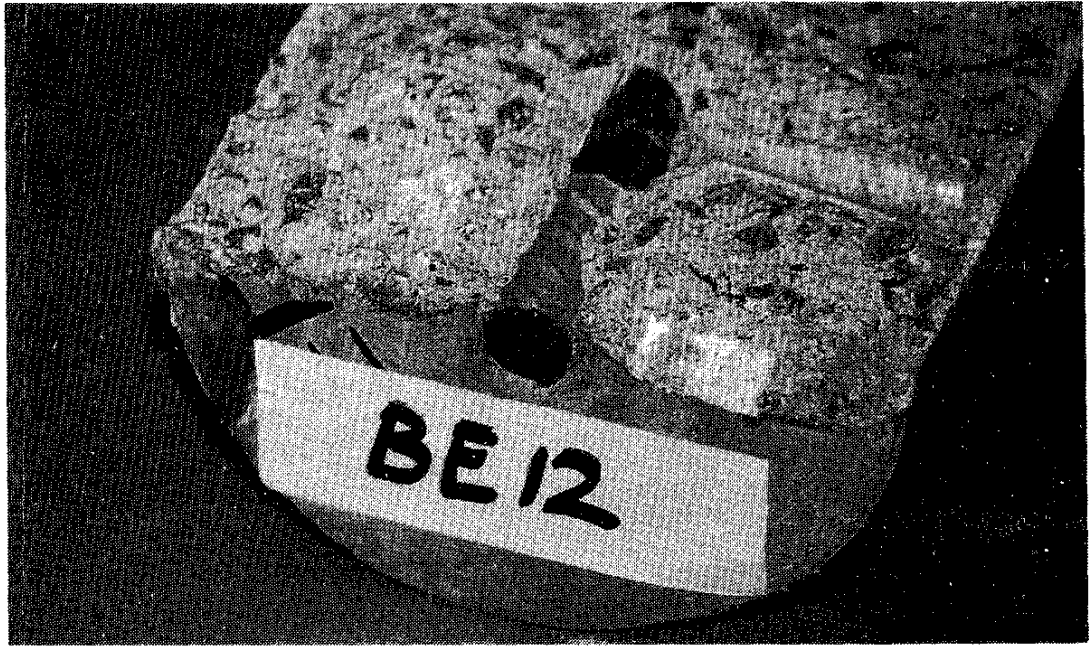
Plate 11: Sample BE12: Epoxy Coated - Salt Fog - 132 Days. General corrosion at unrepaired exposed end of longitudinal bar.
