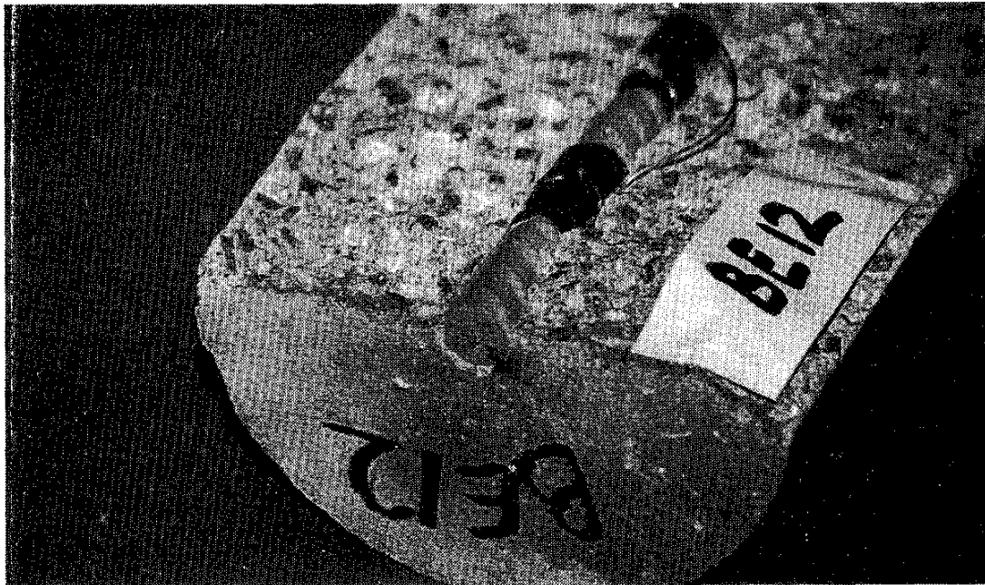
Plate 10: Sample BB12: Epoxy Coated - Salt Fog - 132 Days. Localized corrosion at repaired exposed end of longitudinal bar.
