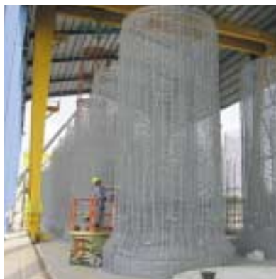
Deep Tunnel Sewage System, Singapore
