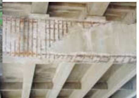
Effect of corroding reinforcing steel
