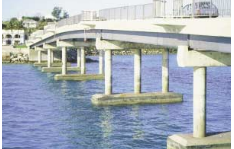
New Watford Bridge, Bermuda
