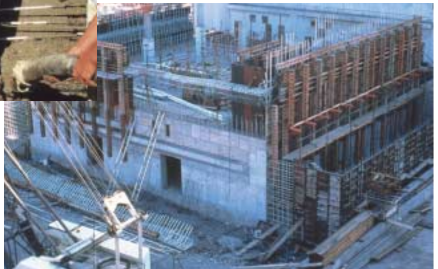
Steelworks - coke ovens storage
