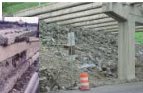
Effect of corroding reinforcing steel
