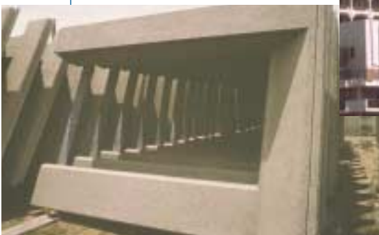
Precast window panels
