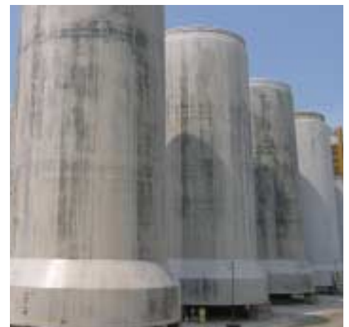
Deep Tunnel Sewage System, Singapore
