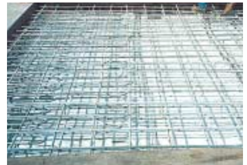
North American bridge decks
