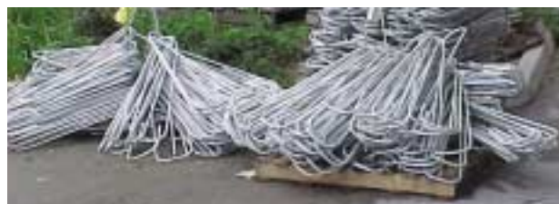
Galvanized rebar stored at job site
